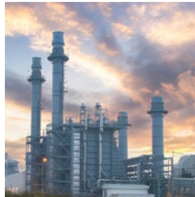
Combined Cycle Power Stations
